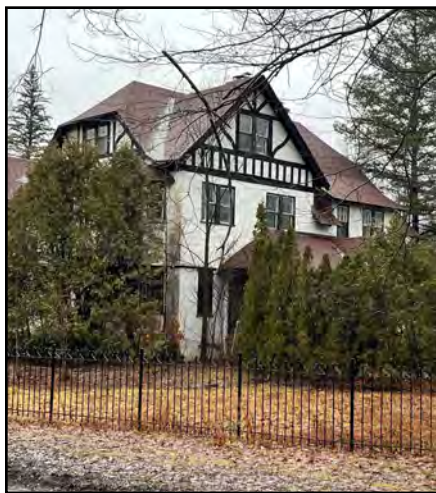
1 Maple Lane awaiting demolition.
