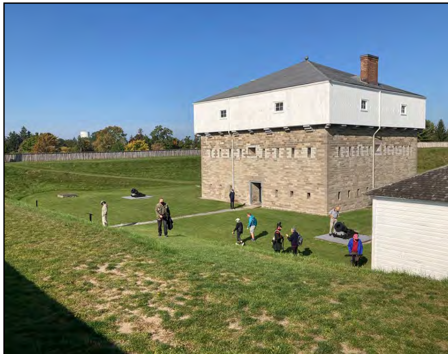
Fort Wellington at Prescott, watching over the St. Lawrence River across from the USA.
