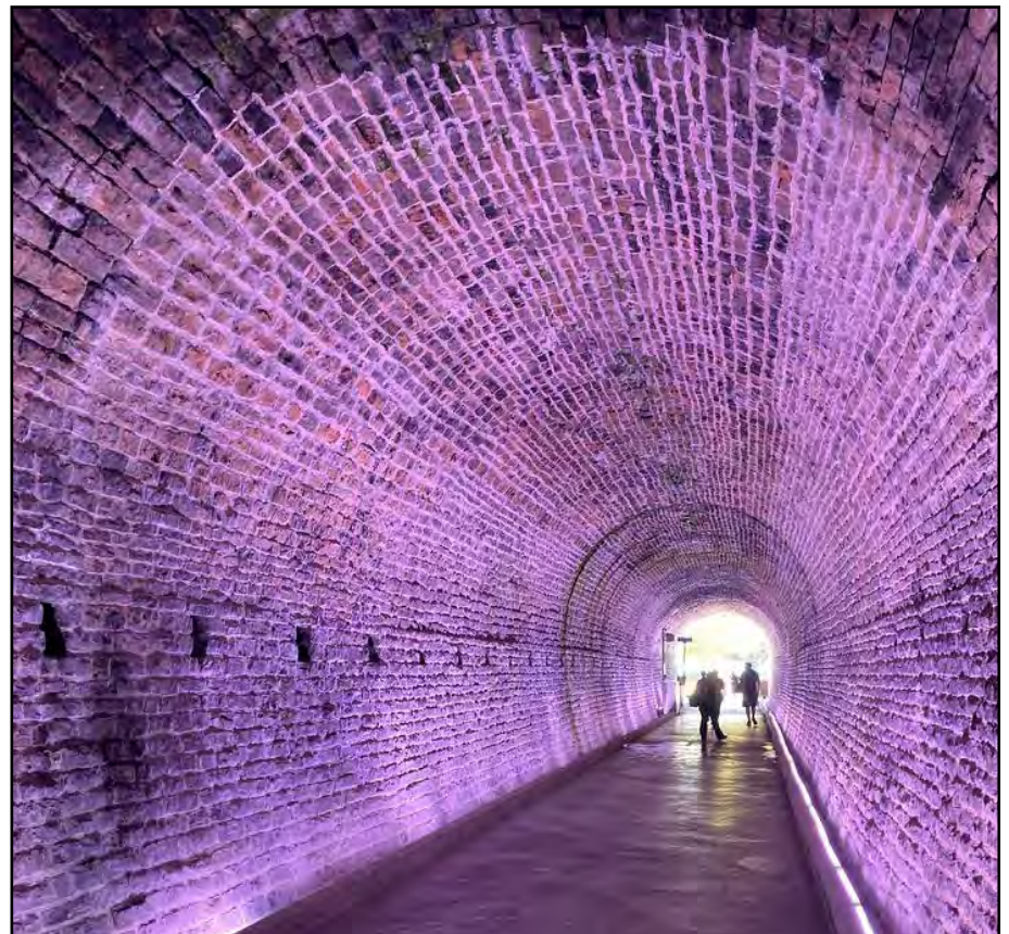
Inside the Brockville Railway tunnel.
