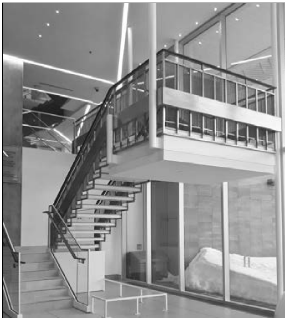
The modernist staircase from the Firestone house on Minto Place now incorporated in the new Ottawa Art Gallery
