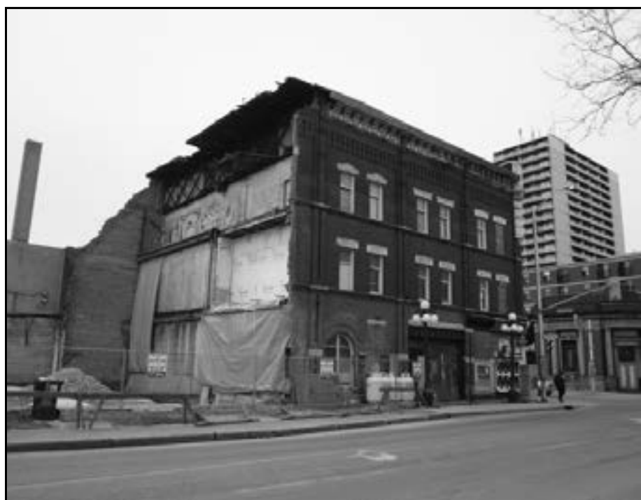
Rear of Somerset House from Somerset Street
