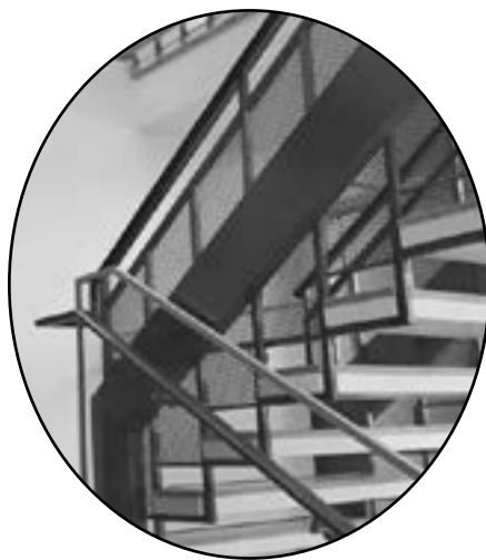
Detail of the modernist Firestone house staircase in its new home.
