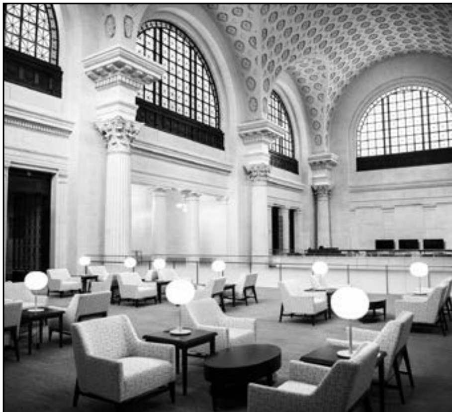
A new mezzanine level added to the grand former waiting room with the massive cast-iron Diocletian windows restored.
