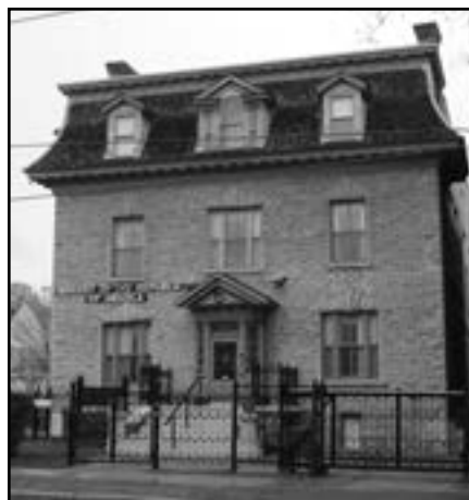
189 Laurier Avenue East (Panet House) 1989 Award of Excellence Adaptive Re-use
