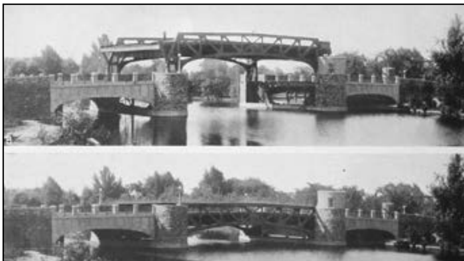
Pretoria Avenue Bridge 1934
