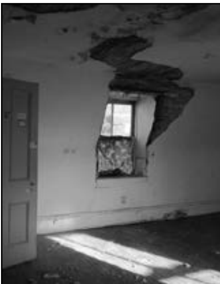
Simard House prior to renovation – upstairs room
