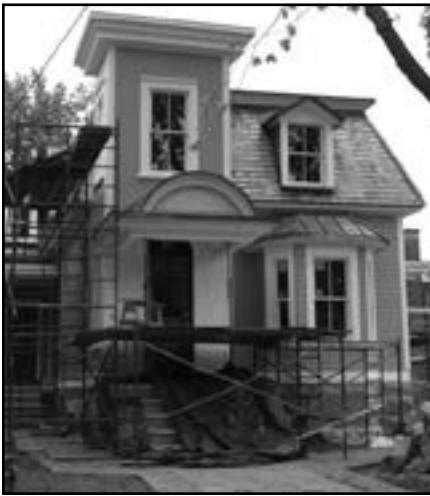
Simard House during restoration
