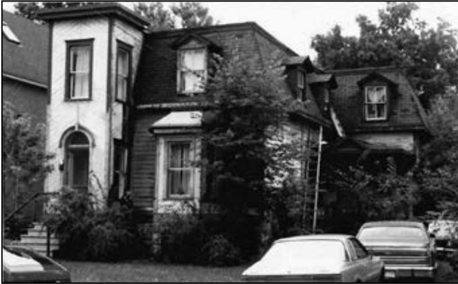
Simard House – maintenance urgently needed
