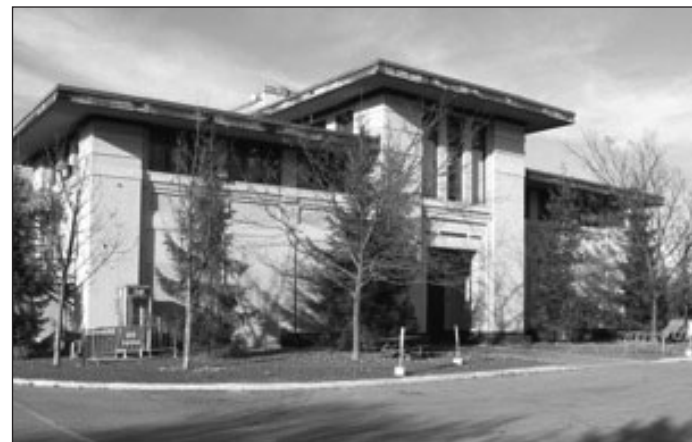
The Horticulture Building, a structure of substantial size, may suffer serious damage if moved.
