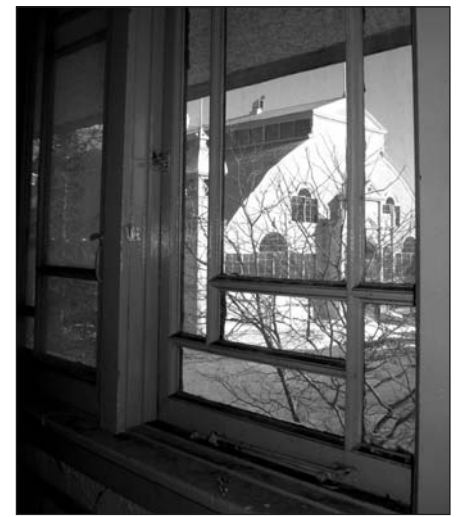
The view from a window of the Horticulture Building shows its proximity to the Aberdeen Pavilion. The proposed move will alter the historic relationship between the two.
