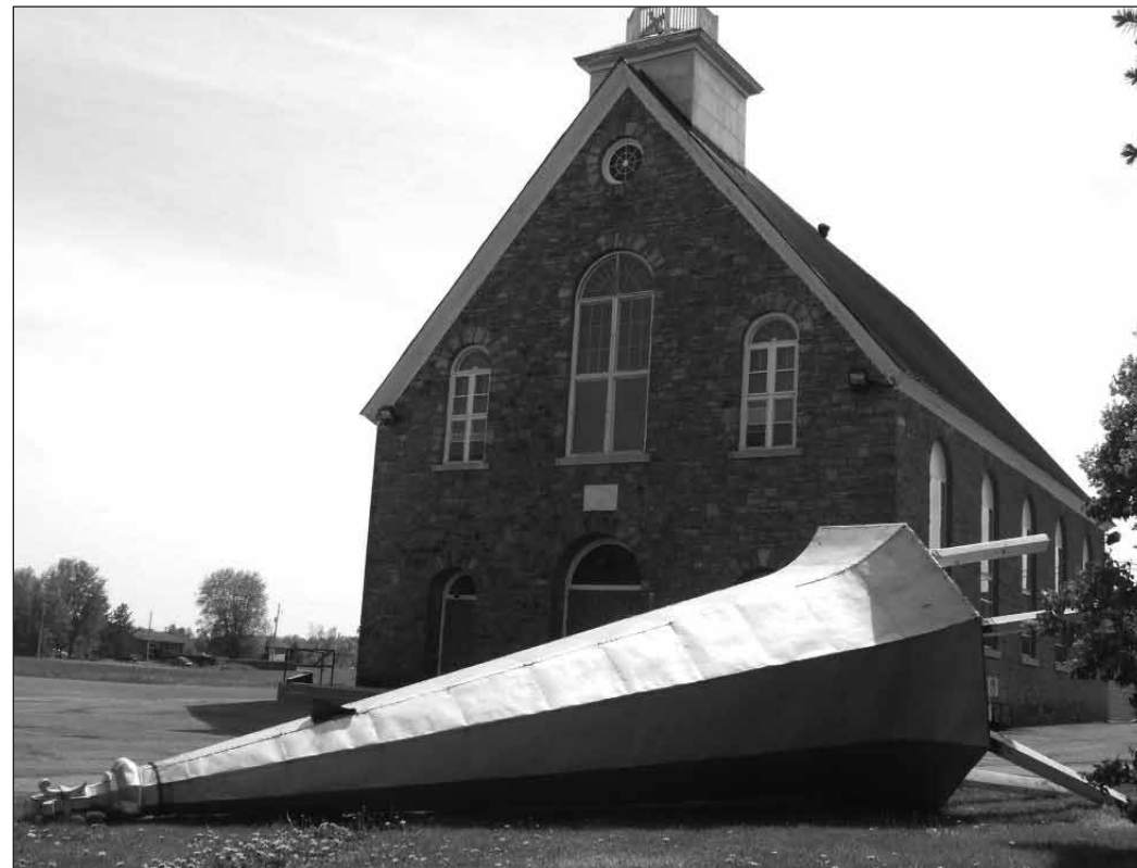
Principal elevation of St. Isidore Church with demolished steeple, June, 2009
