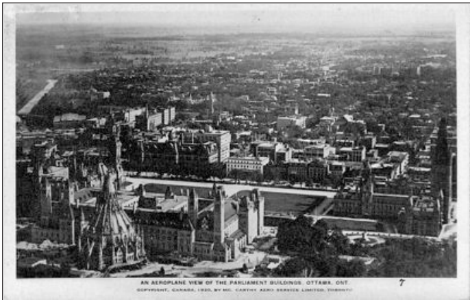
Postcard. Oblique aerial photograph of Parliament Hill from the north. McCarthy Aerial Service Limited, Toronto, 1920
