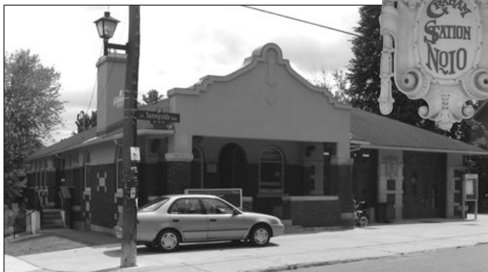
Sunnyside Community centre, formally the #10 Graham Fire Station, is an historic gem in Old Ottawa South.
