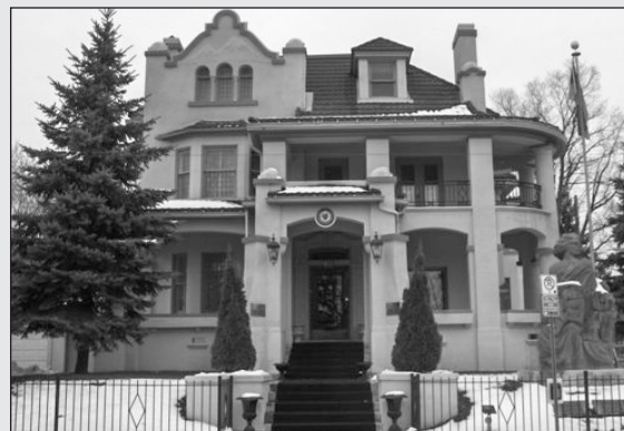
The Embassy of the Republic of Armenia is new to Doors Open and it is housed in a beautiful Spanish Colonial Revival style mansion at 7 Delaware Avenue in Ottawa. W. E. Noffke remodelled the mansion in 1922 and the exterior walls were redone in honey-beige stucco. It’s quite impressive, inside and out.
