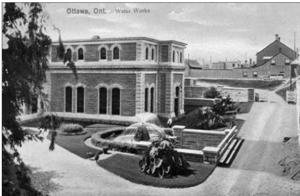
Postcard c. 1907 with a view of the Fleet Street Pumping Station 1874-75. The original Mansard roof had been replaced by a second storey in 1899.
