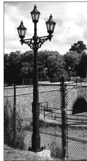
This decorative light standard outside the Fleet Street Pumping Station was reproduced in the 1990s from an original design used on the Minto Bridges.
