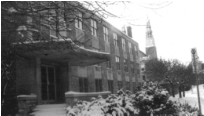
90 Parent looking west on Guigues and concealing 60 Guigues.
