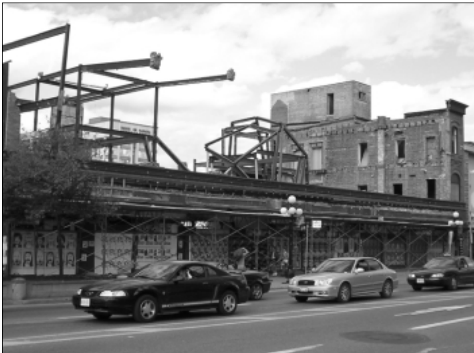
Caplan building under demolition.
