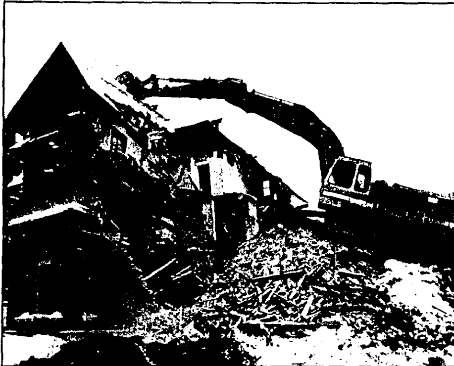
191 and 215 Somerset West: demolished in mid-January
