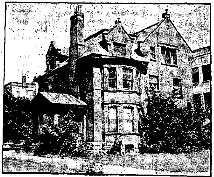
215 Somerset (left) and 191 Somerset (above) were demolished in mid-January to make way for a 40-unit condominium
