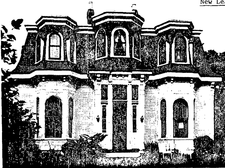
One of Newfoundland's older buildings, lovingly photographed by Hellmut Schade
