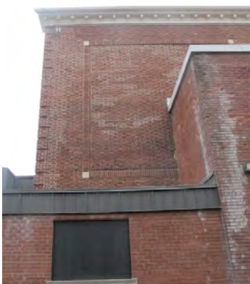
Efflorescence traces, 2012 (Lafontaine & Soucy).
