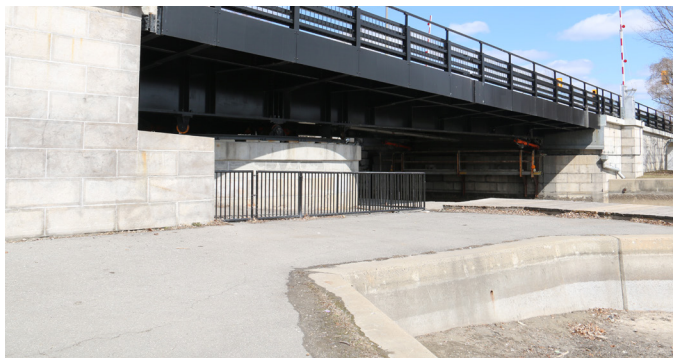
Hogs Back Swing Bridge, 2024. Credit: Matrix Heritage
