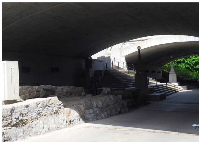
Remains of Sappers' Bridge under Plaza Bridge, 2024. Credit: Matrix Heritage
