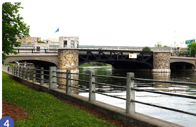
4 View of the Pretoria Bridge.
