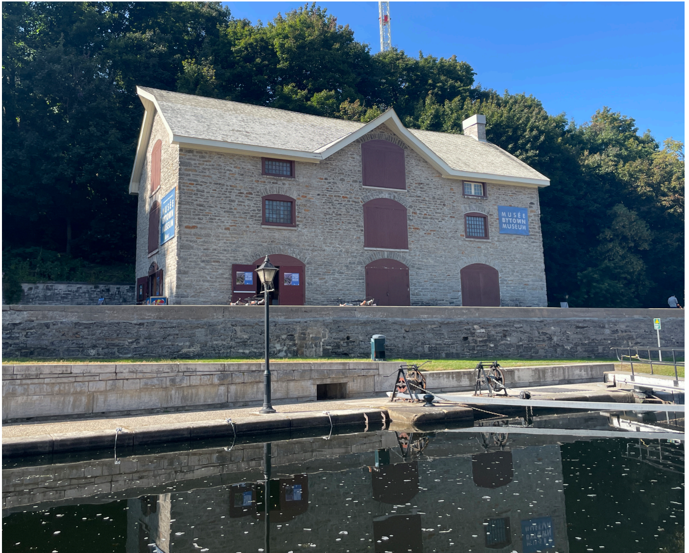
Commissariat Building / Bytown Museum, September 2023. Credit: Matrix Heritage
