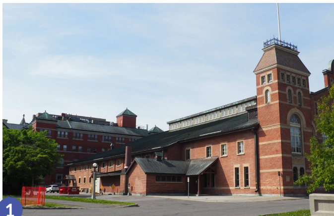
1 View from the Canal and parkway of the row of major turn-of-the-century institutional buildings on the west side of the Canal – Drill Hall, former Military Stores Building, and Lisgar Collegiate Institute.
