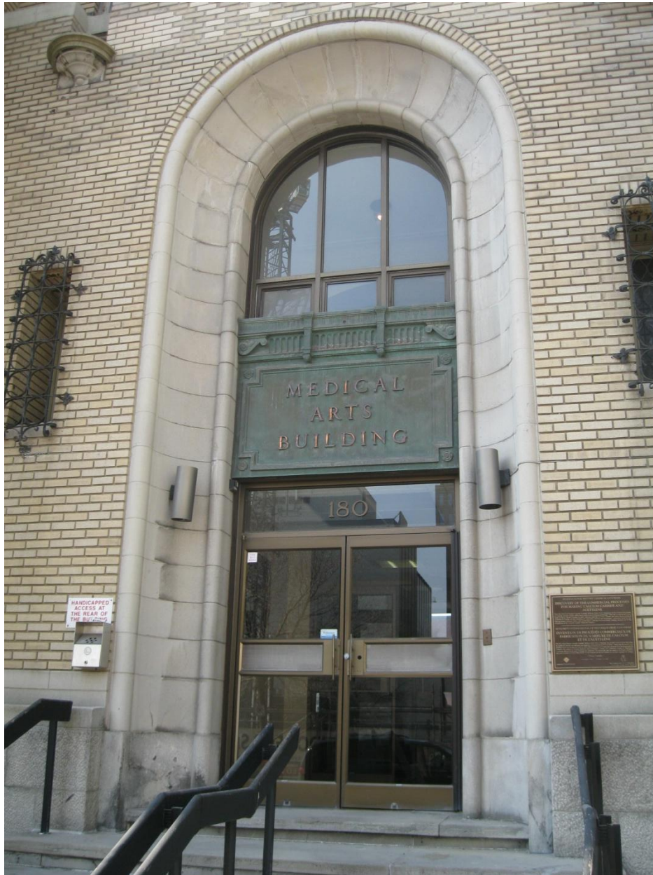
Front entrance of the Medical Arts Building showing limestone door surround and copper frieze above door.
