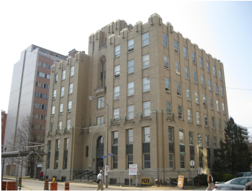
East (front) and north facades at corner of Metcalfe and Nepean Streets
