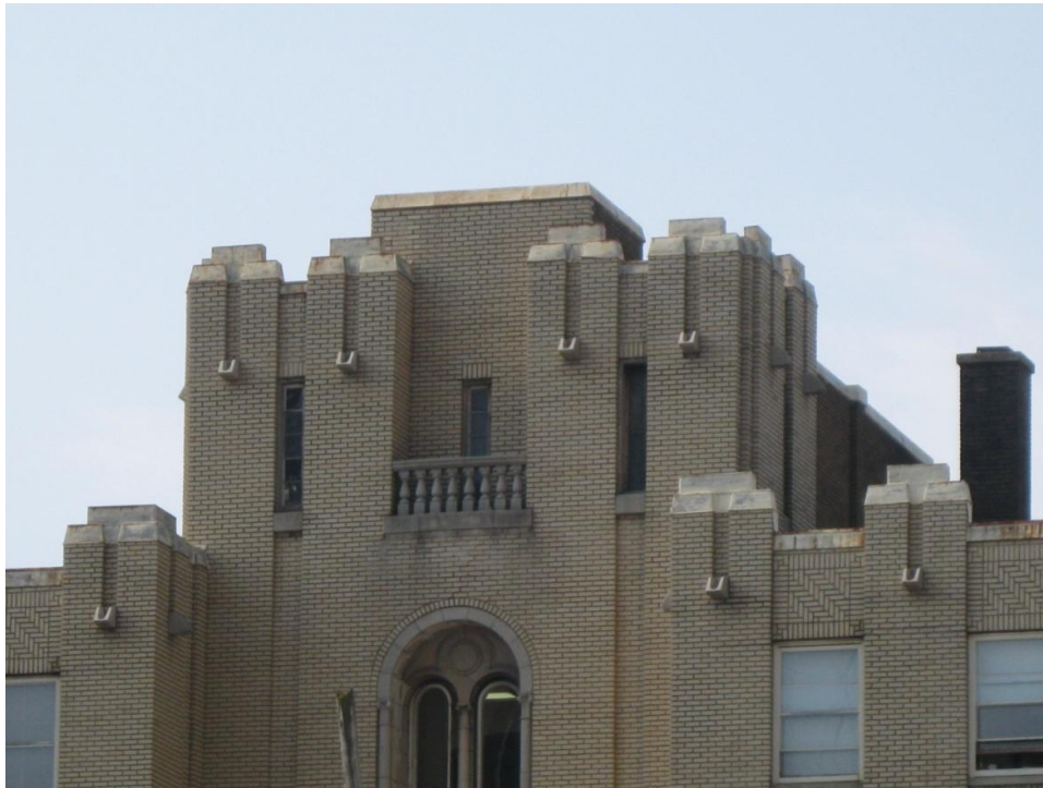
Detailed view of the brick piers that break the roofline and the seventh storey balconet with stone balustrade
