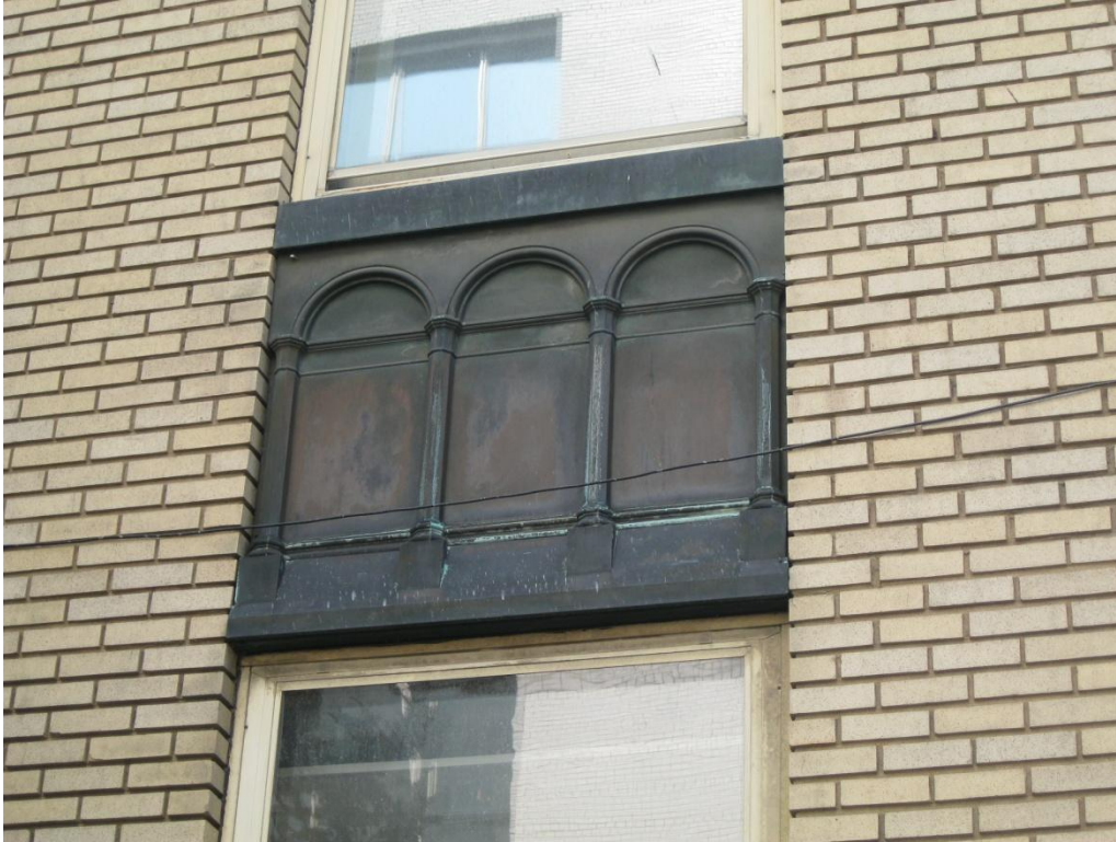
Copper panel between first and second storey windows
