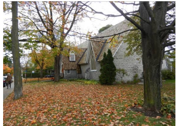
St. Bartholomew's Church
